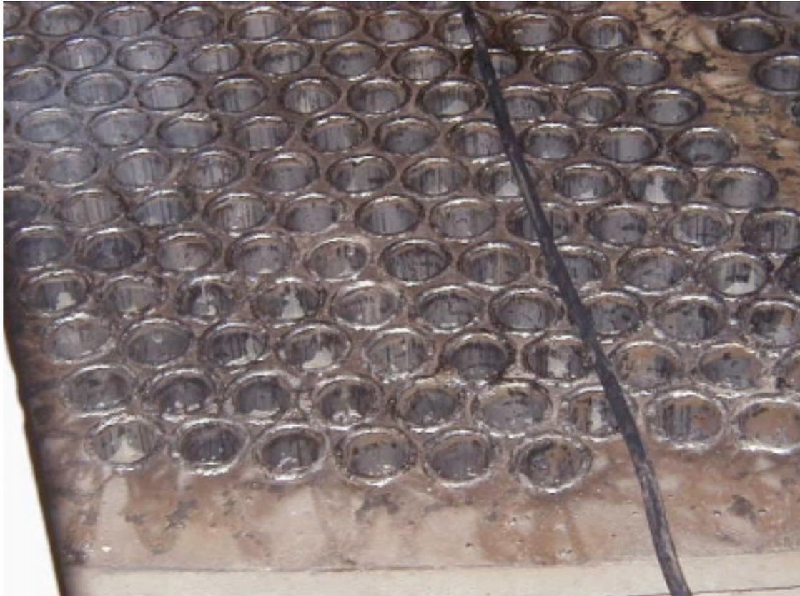
After the introduction of HydroFLOW in the system the heat exchangers and evaporators, remained free of deposits as illustrated in the photo above.
