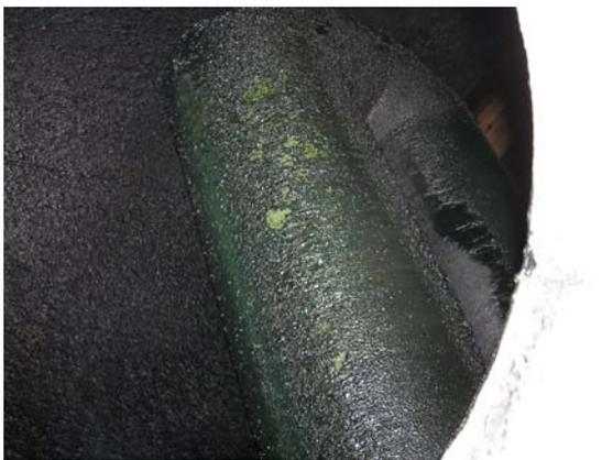
Figure 14 No scale on fire tube
