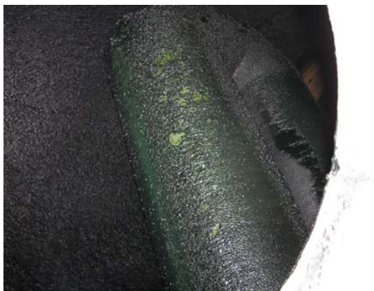
Figure 14 No scale on fire tube
